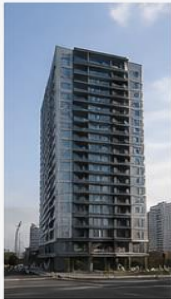
Base-isolated building in Sendai
